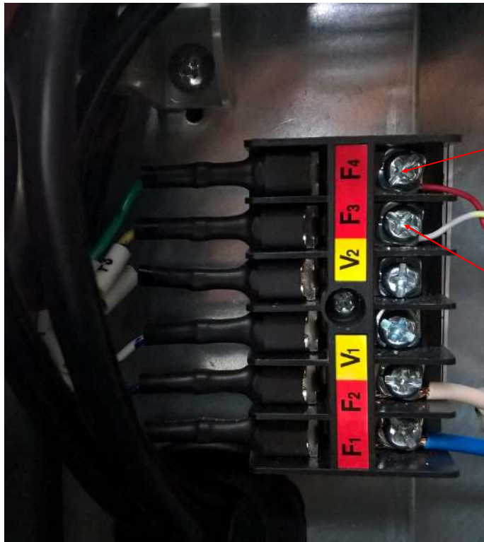
Fig (F) - Samsung indoor fan coil unit terminals
